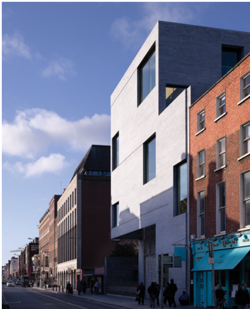
7.7 - The new building of Department of Finance was coordinated by OPW Architectural Services, lead by the Irish State Architect, in Dublin, Ireland (2009); Design: Grafton Architects / OPW Architectural Services; (source: DG - Denis Gilber)
