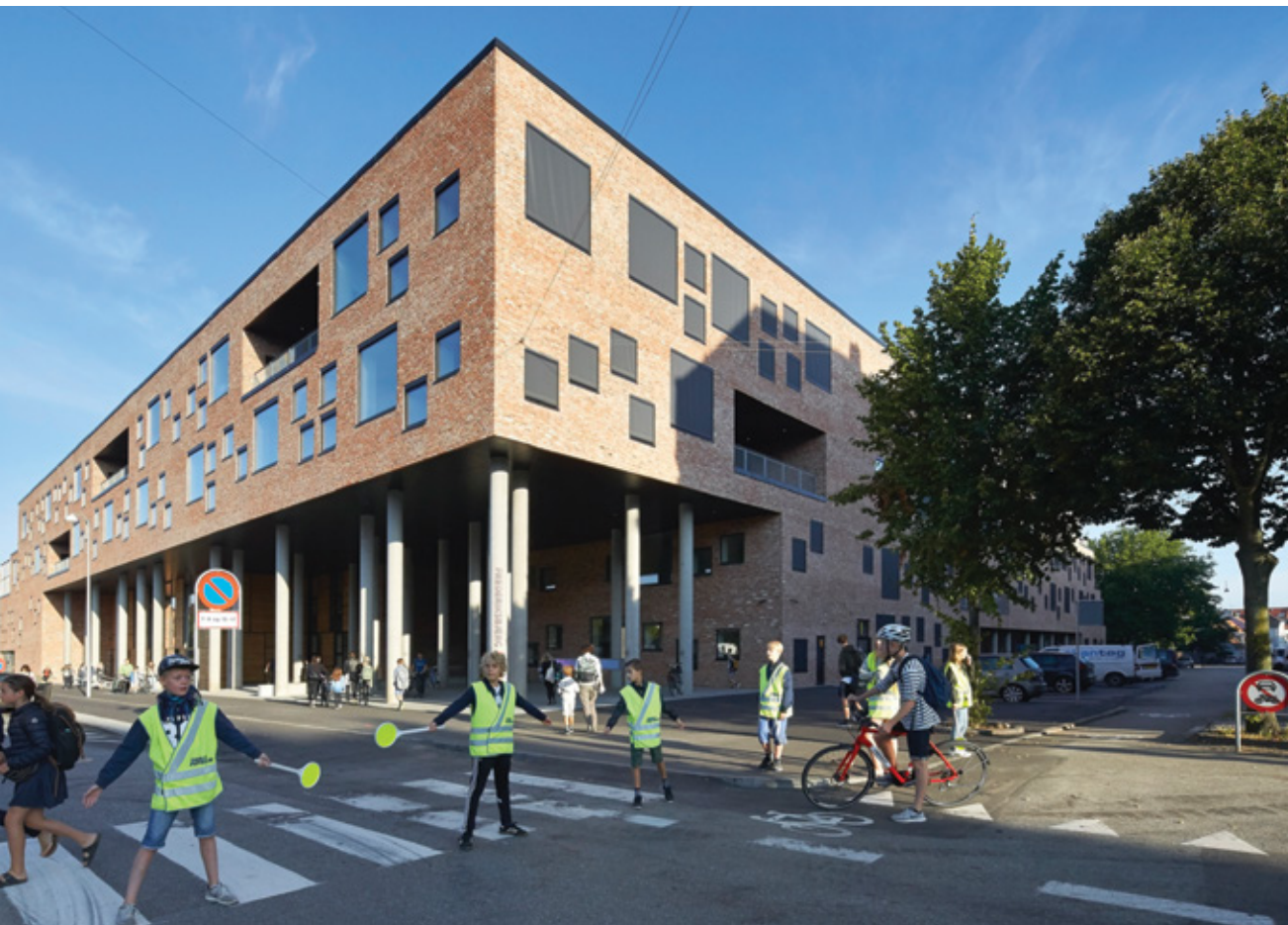
7.9 - The new Frederiksbjerg high school, in Aarhus, Denmark, Designed by Henning Larsen Architects, 2016 (source: Hufton + Crow)
