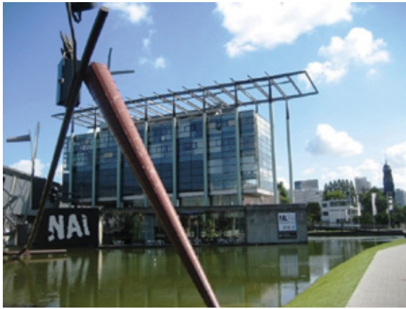
5.9 - The Netherlands Architecture Institute (NAI) opened in 1993, following the merge of three architectural cultural organizations some years before, designed by Jo Coenen & Co; now is part of The New Institute (Het Nieuwe Instituut), Rotterdam (source: F.Eveleens).
