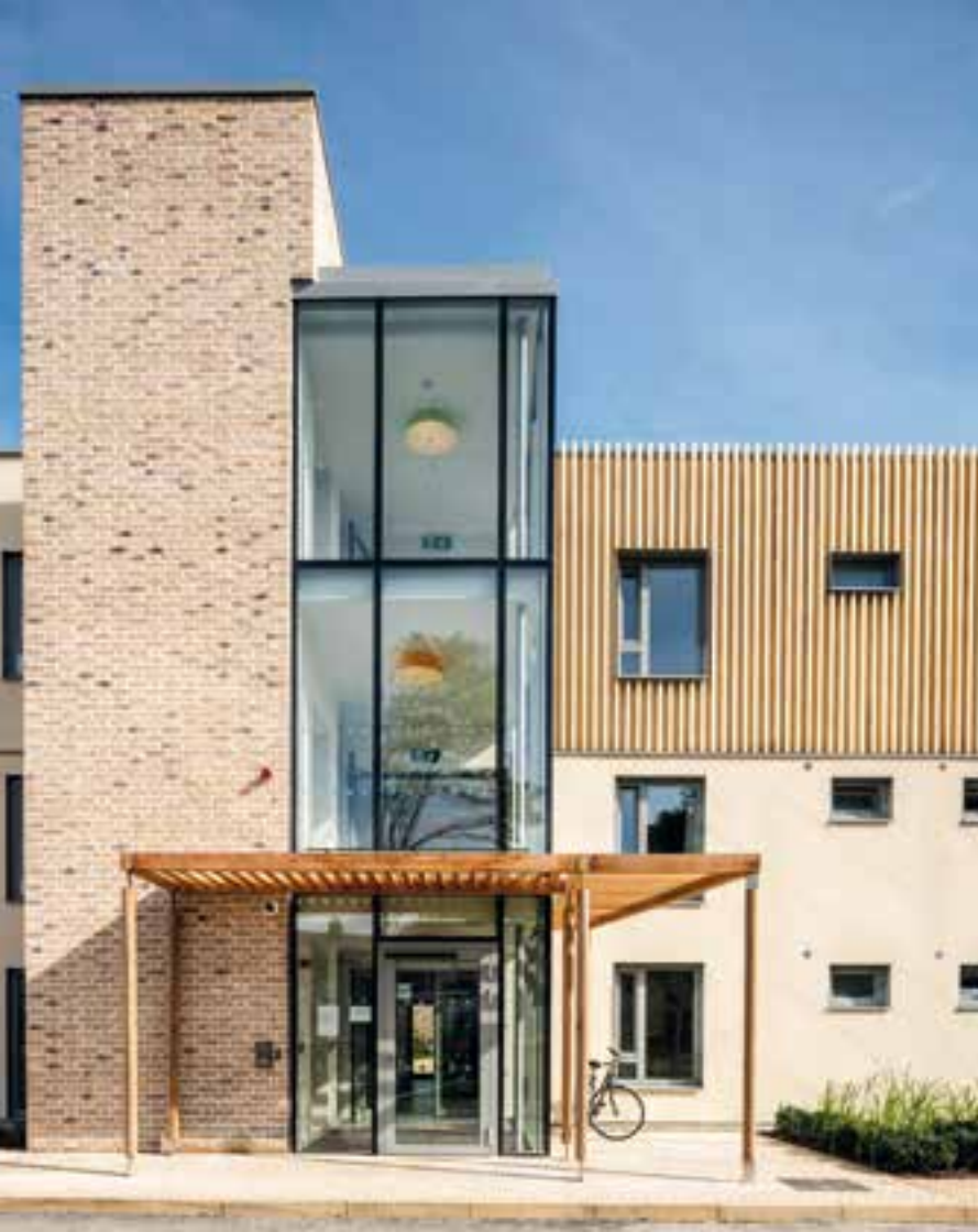
Loc.: Sallynoggin, Co Dublin (Ireland / Irlanda) Arch.: Dún Laoghaire Rathdown County Council Architects Department Y.: 2016 A.: HRIA Awards - Sustainable Project (2017) Cert: EnerPHit
