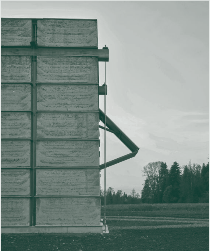
Kiln Tower in Rammed Earth, Cham, Switzerland
