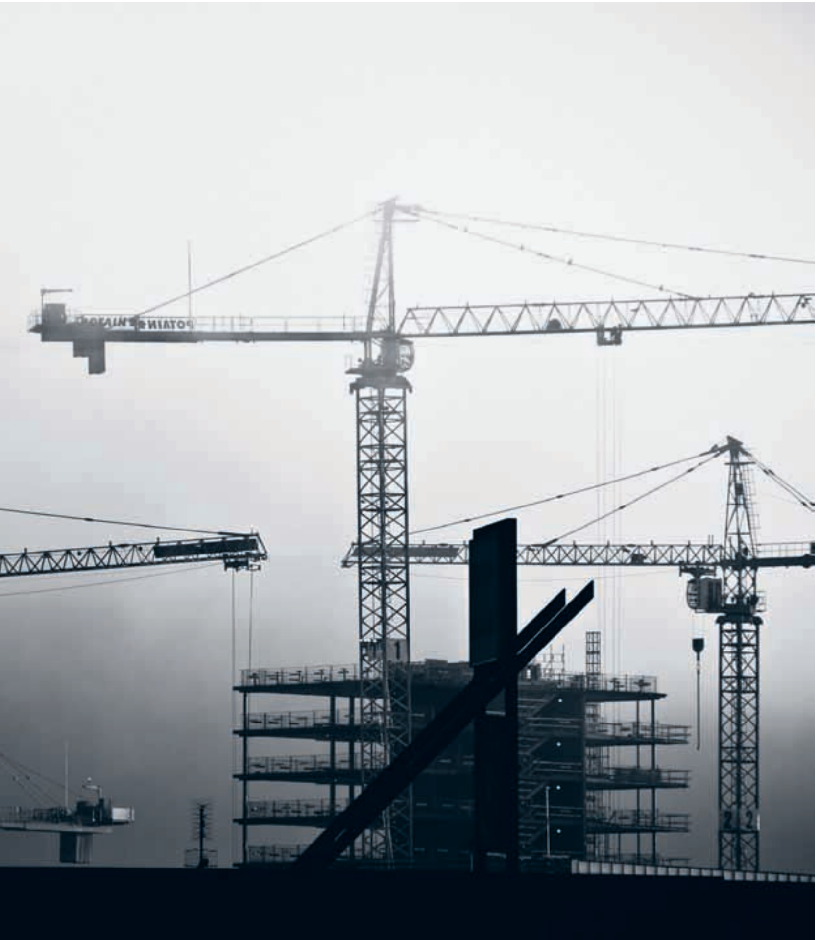
[0.7] Building site. Bjørvika, Oslo
