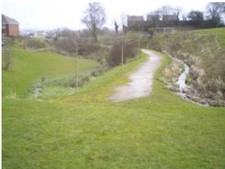
39 Sustainable drainage systems at Pontyclun
