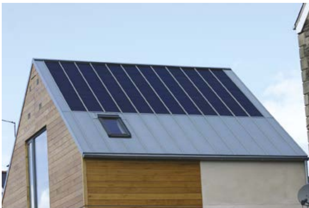
21 | Solar panels, Coach House, Cardiff
